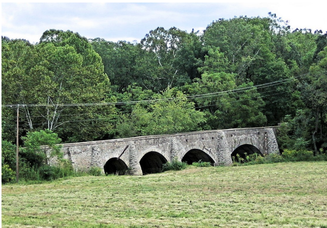
Goose Creek Bridge (Jim Lewis)
