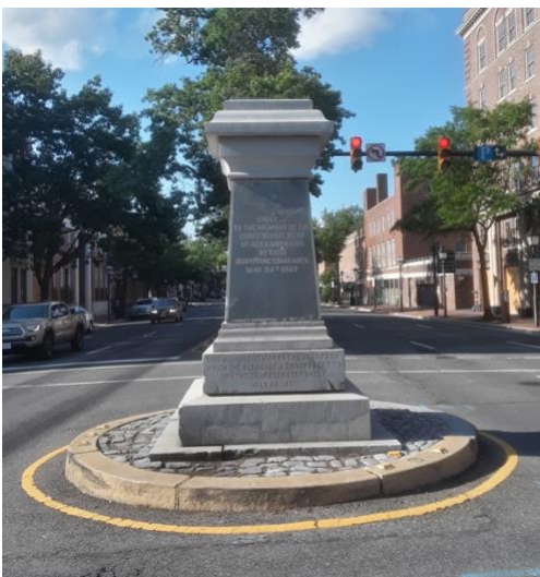
Pedestal After Removal of Appomattox Statue June 3, 2020
