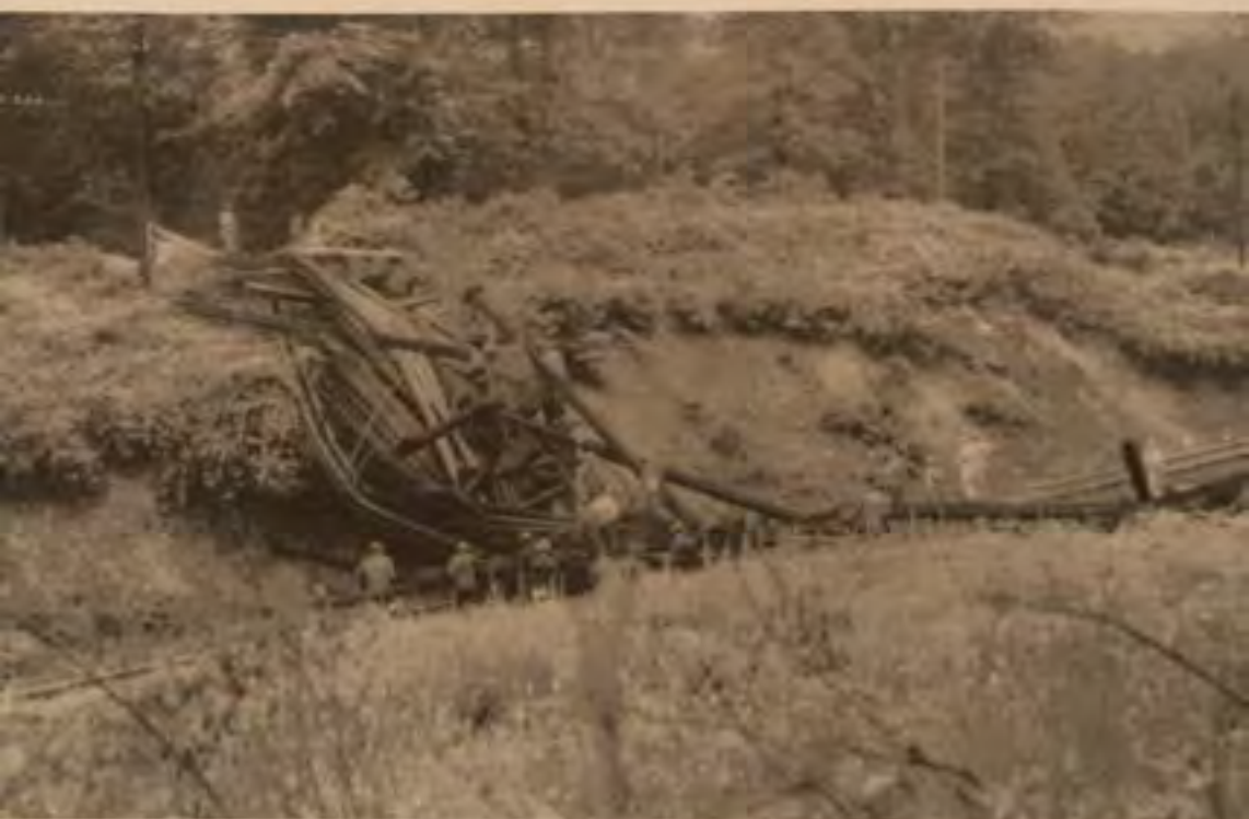
iron truss bridge was built by the company after 1894 the traffic on Ox Road over the Southern Railway of right-of-way. It collapsed early on the morning of
