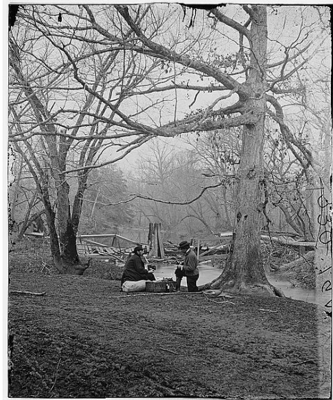
RUINS OF THE RAILROAD BRIDGE FORMERLY ACROSS BULL RUN
