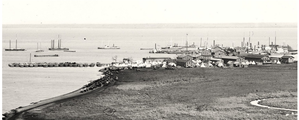
Aquia Creek Supply Depot
