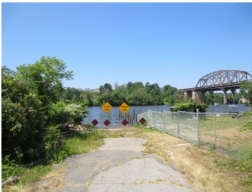
Current view of Old Colchester Rd. approaching its old Ferry Landing
