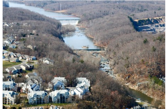
Aerial photo of both dams on the Occoquan Reservoir
