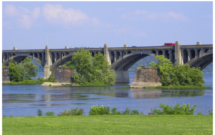
Wrightsville Bridge today (Janet Greentree )
